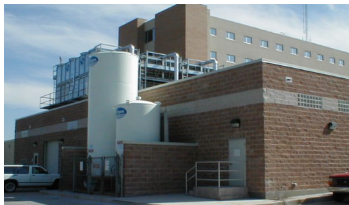
DEACONESS HOSPITAL CENTRAL PLANT, Oklahoma City
