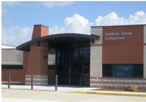
ARDMORE ELEMENTARY SCHOOL, Ardmore
