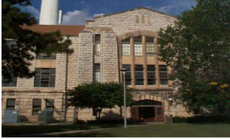
KSU CHILLER PLANT, Manhattan, KS
